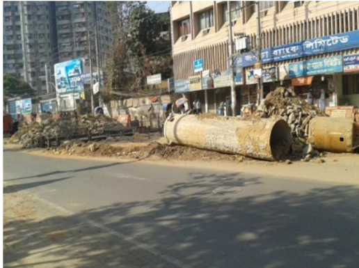
Figure 3a. On street construction in Moghbazar, Dhaka (May, 2015).
