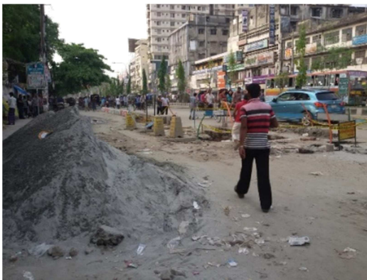
Figure 3b. On street construction in Moghbazar, Dhaka (May, 2015).
