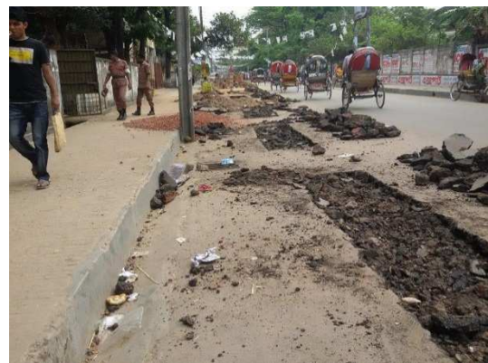
Figure 2. Construction work in Dhakeshwari Road.
